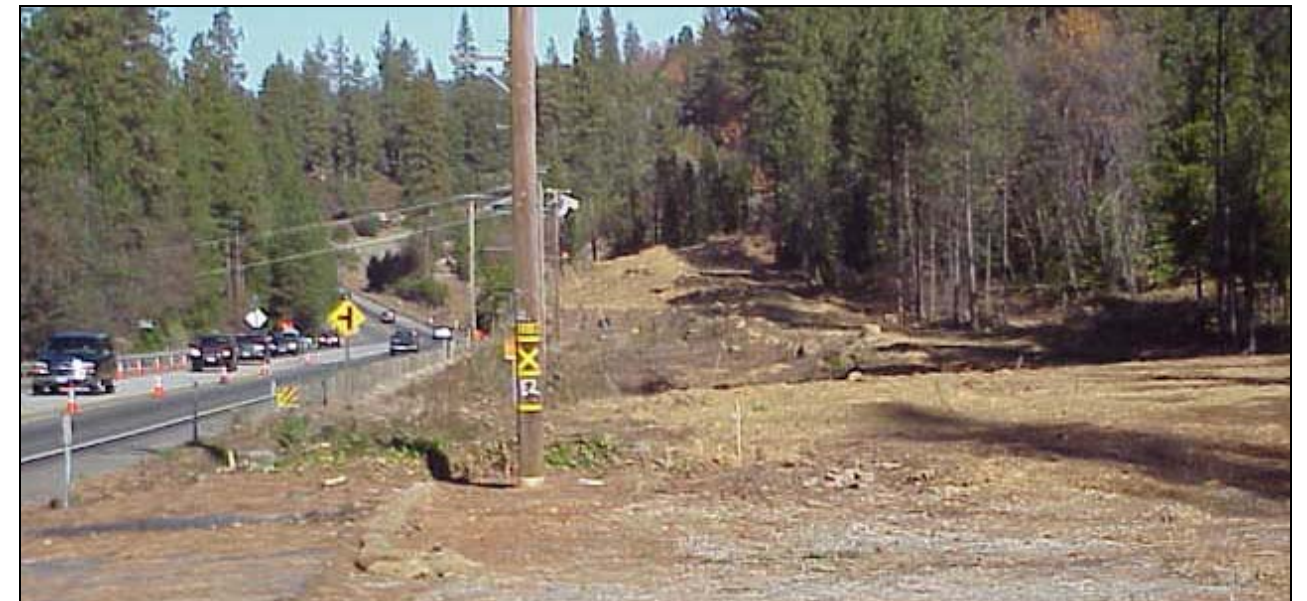
Tree removal on SR 49 just north of La Barr Meadows Road where the four lane highway and shoulders will be constructed.
